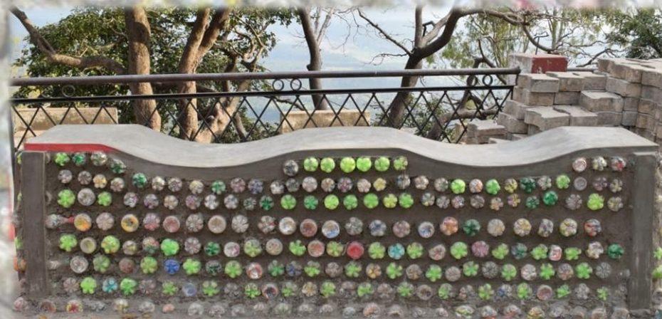
POLY BRICK BOUNDARY WALL
