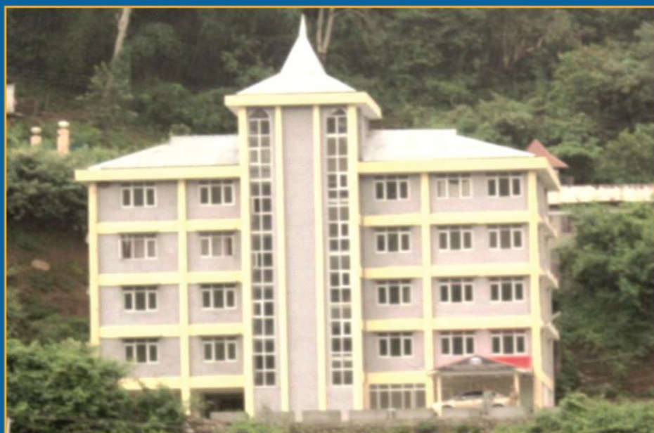
A Complex of RFSL, CR, Mandi, (Front view)
