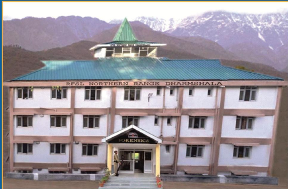
A Complex of RFSL, NR, Dharamshala, (Front view)
