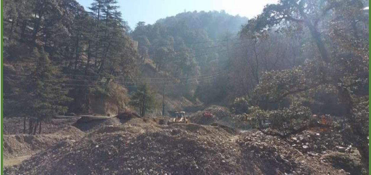
Figure 1: Project site during initial construction of new OPD block
