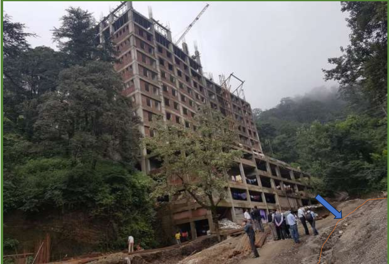
Figure 2: Proposed land during new OPD building construction
