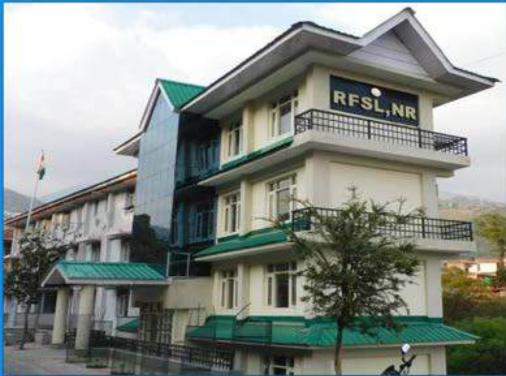
A New Complex of RFSL, NR, Dharamshala
