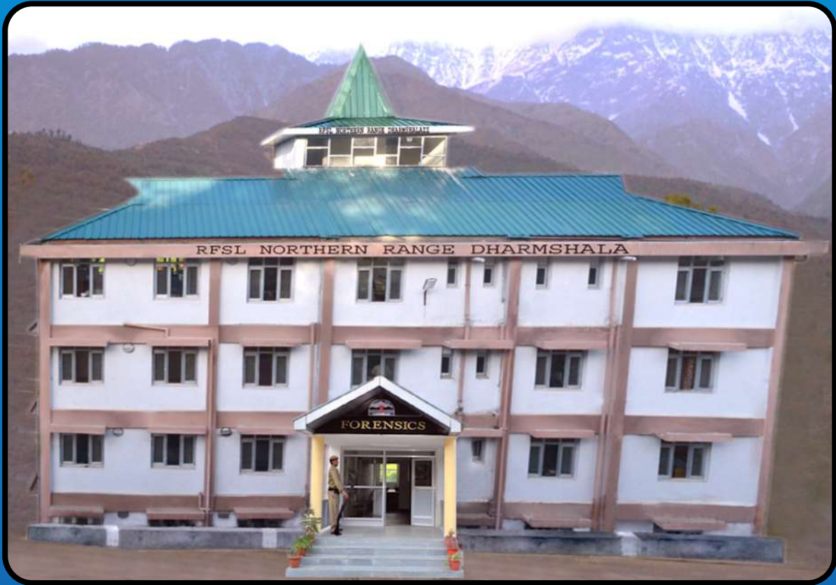
A Complex of RFSL, NR, Dharamshala, (Front view)
